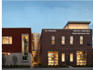
2011 Merit Award Winner: City of Minneapolis Hiawatha Maintenance Facility
