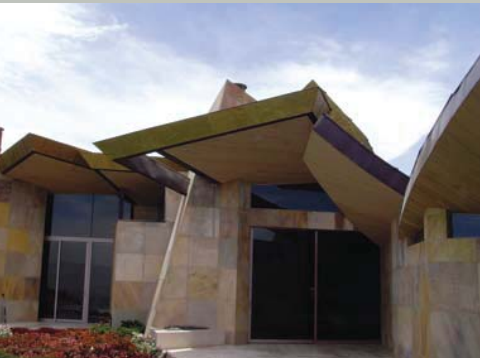
Duane Hagadone's 32,000-square-foot mansion in Palm Desert, Calif., gets its unique look from its custom gold crystal finish titanium fascia and 20-ounce TECU Oxide coated standing seam panels. (Photo courtesy of MG McGrath Inc.)
