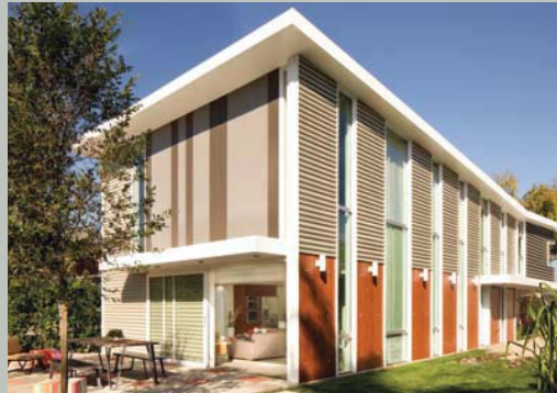
Depending on the desired effect, designers may choose from a variety of materials including copper, stainless steel, coated aluminum or coated Galvalume exterior metal wall panels for luxury residences. (Photo courtesy of Metal Sales Manufacturing Corp.)
